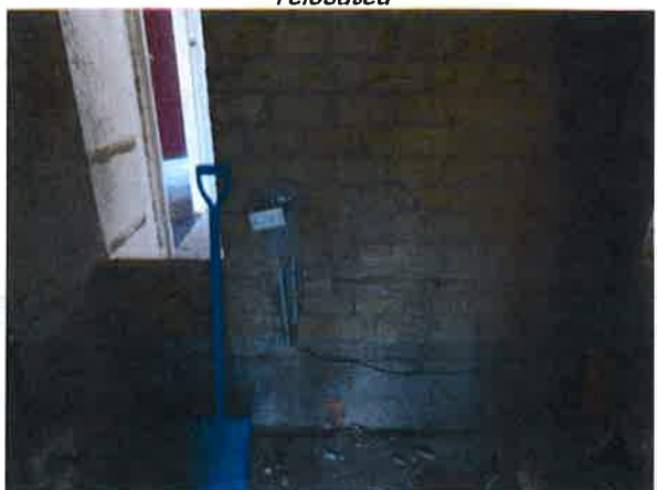
Figure 12: Photo of the existing bathroom to be enlarged and upgraded
