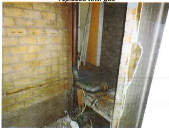
Figure 11: Photo of the existing bathroom to be enlarged and upgraded
