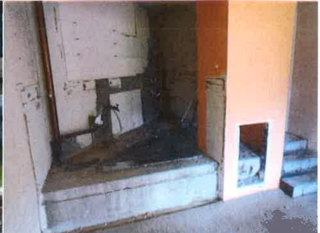
Figure 6: Photo looking from the living area to the kitchen
