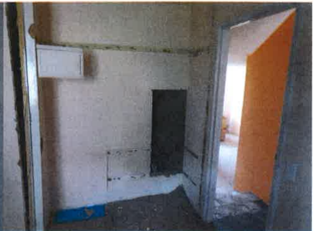
Figure 10 Photo of bedroom two showing door to be relocated
