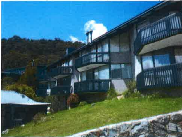
Figure 5: Photo of the exterior of the building
